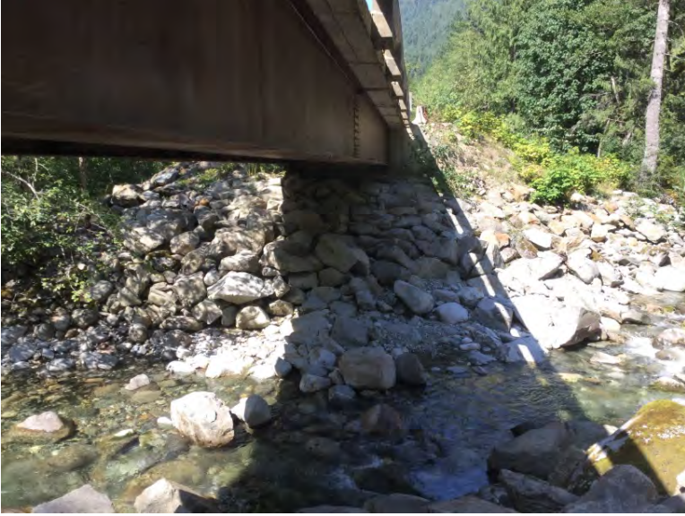
Right Bank Abutment when facing downstream
