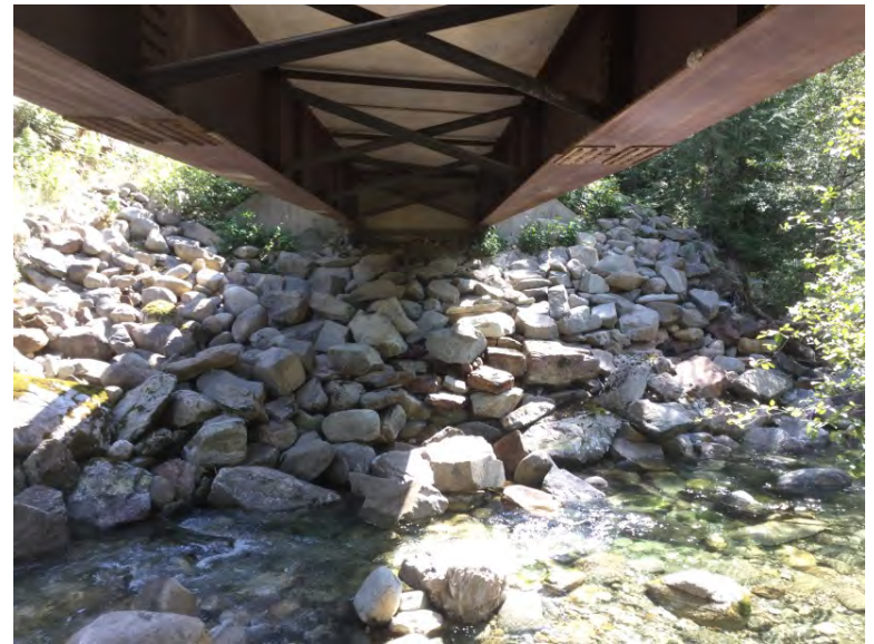
Left Bank Abutment when facing downstream
