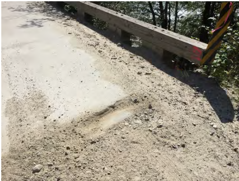
Deck elevation 2 inches higher than ballast walls
